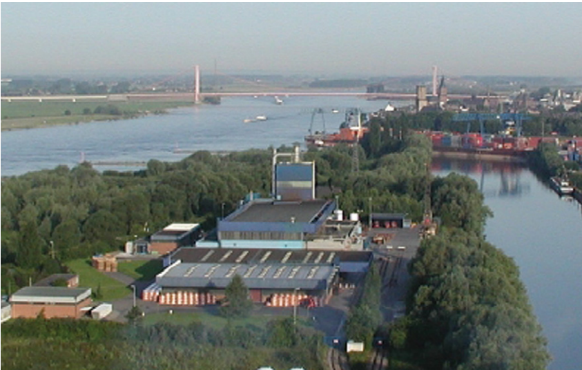
Figure 2. Taking advantage of the production plant's location, water from the Rhine is used for cooling.
