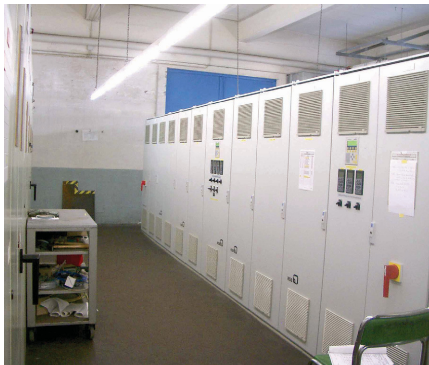
Figure 5. To operate most efficiently, the system comprises two closed loops with two pump control systems for continuously variable speed control, type Hyamaster SPS – this is the control panel.
